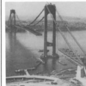
In the case of the colossal Verrazano bridge (whose length has only been surpassed by the Humber bridge in England), the 693 feet towers soar to the height of 60 story skyscraper, the four cables consist of 143,000 miles of pencil-thin wire and the anchorages contain a total of 375,000 cubic yards of concrete.
